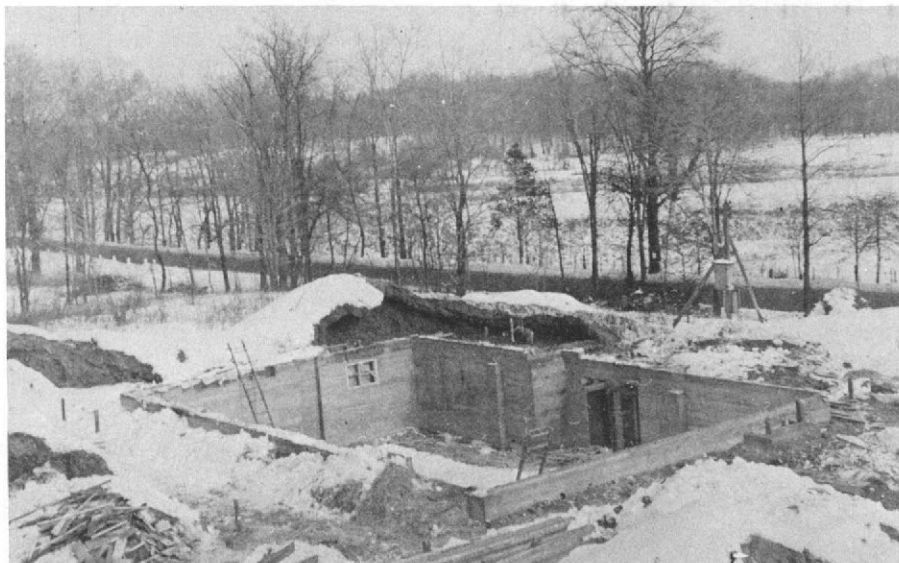
It was a long, cold winter, but work continued on the new building into early 1938.
