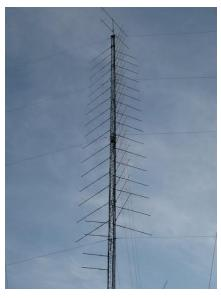
Why were the Grid Pirates (K8GP) loud on 2 meters? 3x16x5ele pointed NE, NW, and SW, plus 4x5ele pointed SE, topped with 2x FO12 rotatable Yagis @ 200'. (Photo by K8GP)
