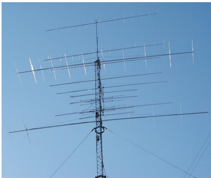
Bob K2DRH put up a new tower this year for his VHF/UHF array made up of 667 elements covering 2 meters through 3456 MHz. (Photo by K2DRH)
