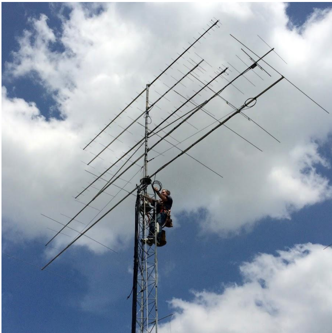
This doesn't look like the "lower" four bands, but George, K5TR, can be seen hard at work getting his VHF/UHF array ready for the contest. From bottom to top (not including George) are seven elements on 50 MHz, 17 elements on 144 MHz, 16 elements on 222 MHz, and a pair of 28-element beams on 432 MHz. [George, K5TR, photo]
