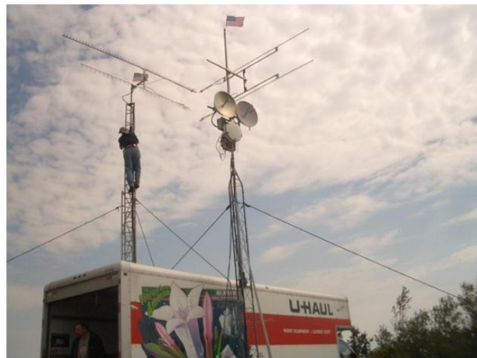
Erecting the microwave station at W3CCX (W3CCX website photo)
