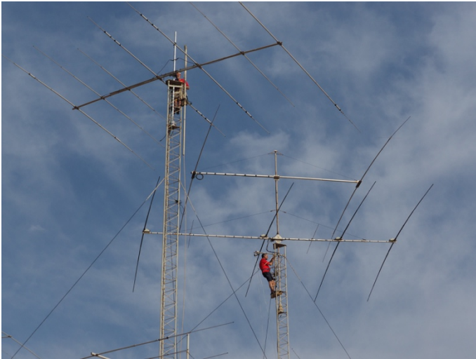
W2GD (left) and DL6RAI (right) performing tower work at P49V in Aruba during the week before the contest. The work was finished just in time for DH8BQA, DL5CW, DL5LYM, DL6RAI to operate the Multioperator, Two Transmitter P40XM together for the first time. [Oliver Droese, DH8BQA, photo]
