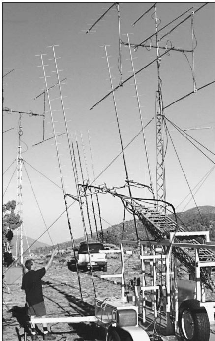
KB6WKT supervises deployment of the 432 MHz and 1.2 GHz arrays at the W6TOI site.
