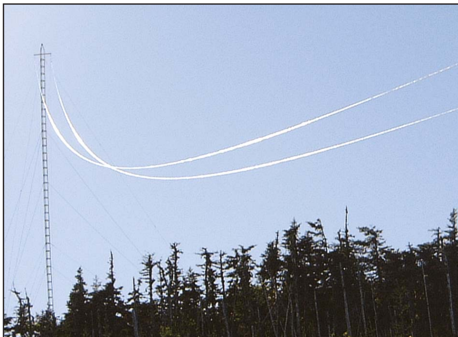
Figure 4—The LF antenna at VO1NA used for several years (including his first transatlantic QSO) consists of two parallel wires 100 meters long, spaced 1 meter apart. The antenna is supported at the far end by a 25 meter tower, and the wires slope down toward another tower near the shack where they are connected together. The antenna is fed at this point with another 50 meters of wire for a total length of 150 meters and matched with the loading coil and variometer shown in Figure 5. The antenna has since undergone several involuntary changes as Mother Nature took down one of the wires and then in January 2005 took the remaining wire and tower during an ice storm. VO1NA is back on LF with 100 meters of wire about 10 meters off the ground. Joe was never very comfortable on the top of his tower and is most grateful he was not there at the time it collapsed. A 30-meter-tall replacement is planned.
