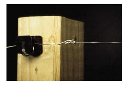
Splices can also create problems, especially if they are between two different types of wire. Splices should be mechanically secure, lessening the likelihood of poor contact, sparking and wire failure.
