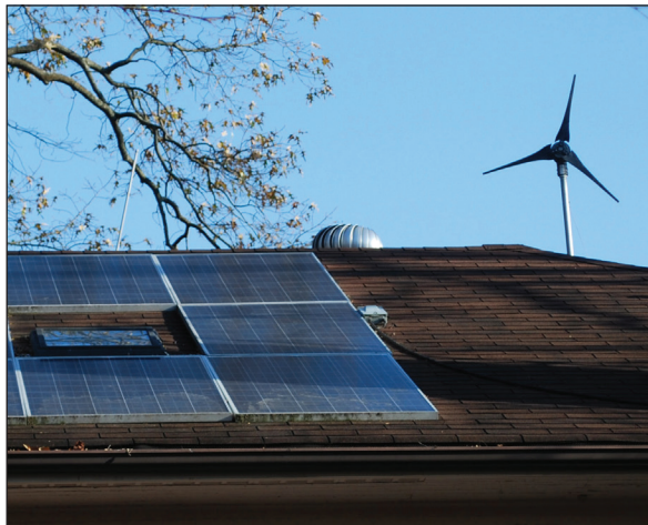
Figure 1.3 — A 4 foot Airpax turbine installed on my roof just to prove how poor home wind is.
