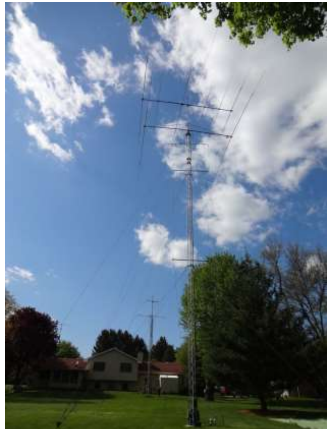
K9MMS towers (K9MMS photo)
