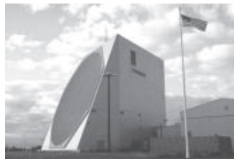
A Pave Paws military radar antenna is actually about 5 stories high and uses the same 70 cm frequencies as Amateur Radio. ARRL has worked to eliminate interference issues while minimizing restrictions on hams.
