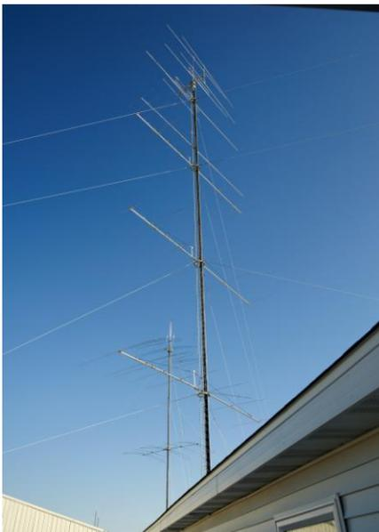
The 10 meter stack and VHF antennas on the rotating tower near the K9CT shack. (Photo KB9UWU)
