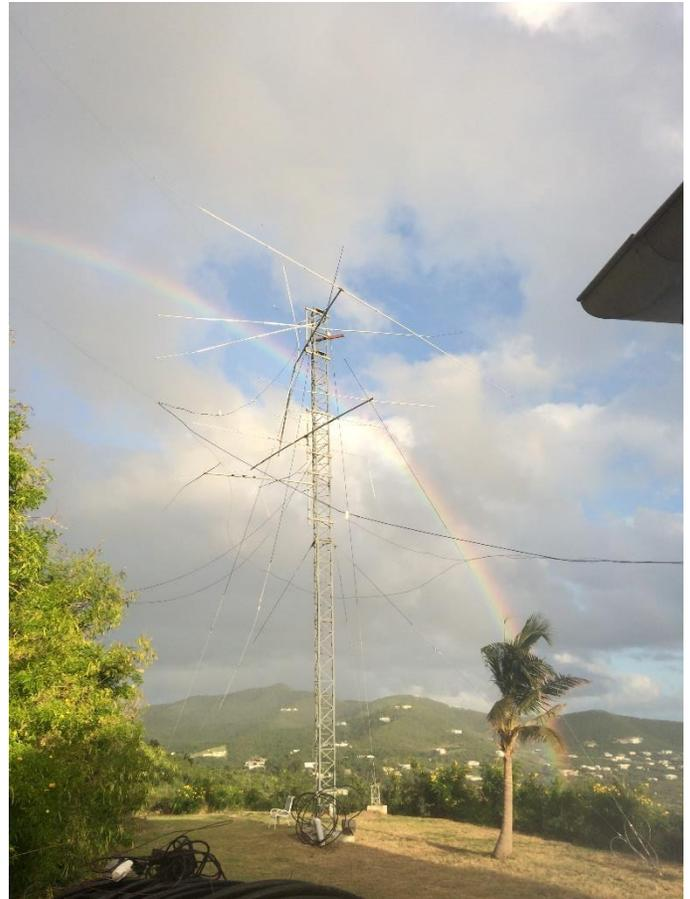
*That's not a new antenna design, it's the aftermath of Hurricane Maria at NP2X. You can't see it here but even the tower has a broken base. Fred, K9VV, estimates wind speed at more than 200 mph. (Photo courtesy — Fred Kleber, K9VV)*
