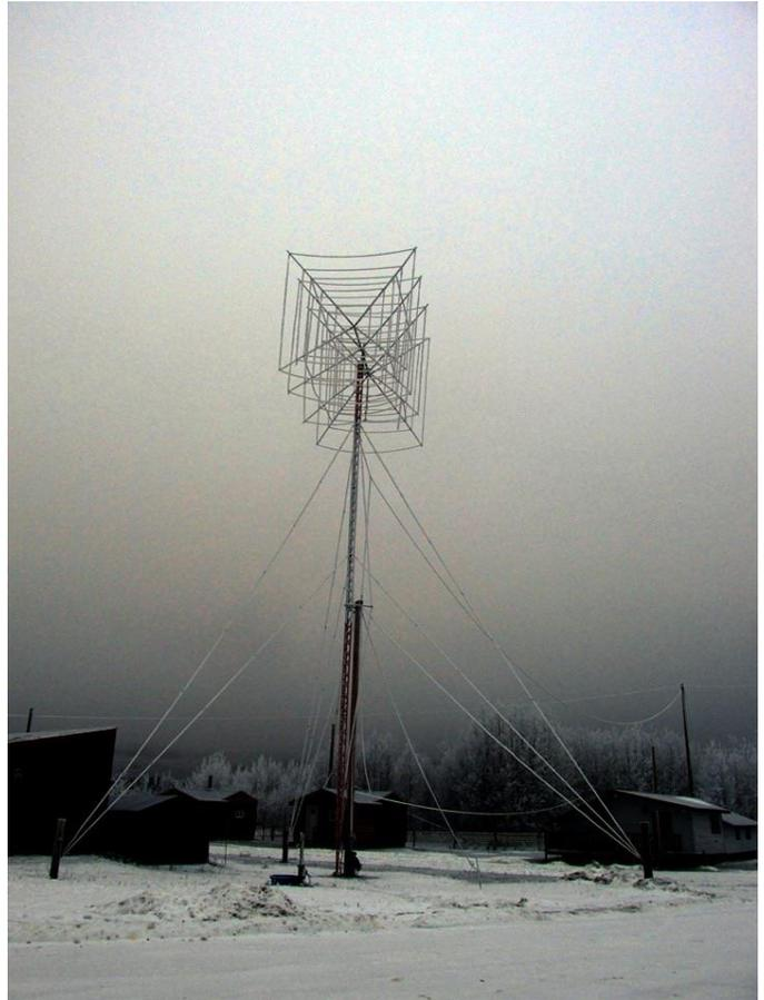
*It's not easy keeping a multi-element HF quad on the air — imagine the challenges in the Yukon! Ice fog coated every inch of the antenna systems at VY1AAA. (Photo courtesy — J Allen, VY1JA)*
