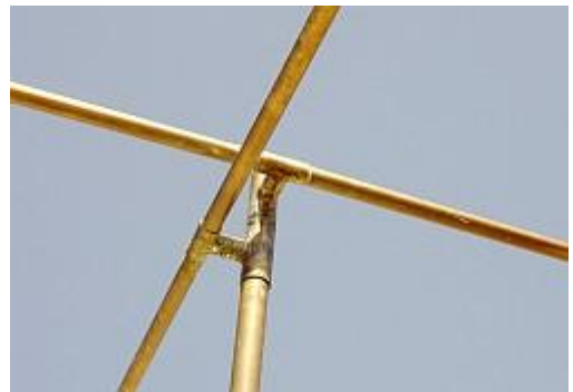
Figure 5 -- Element attachment
