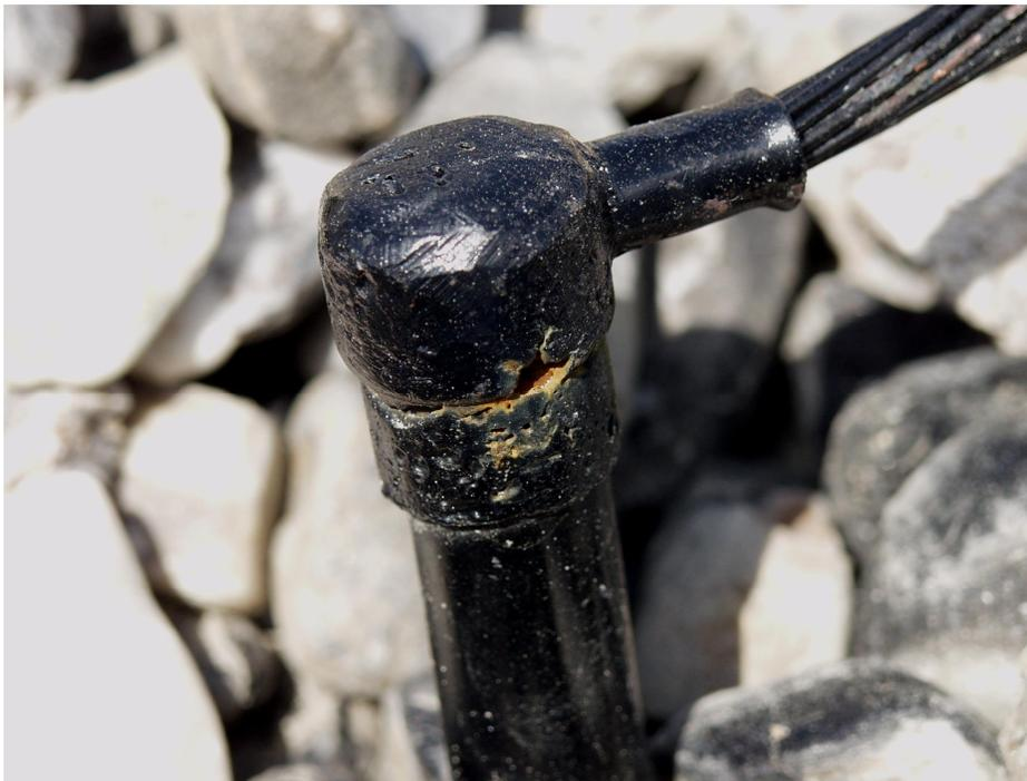
**Figure 15** CADWELD<sup>®</sup> on Antenna Counterpoise Wire
