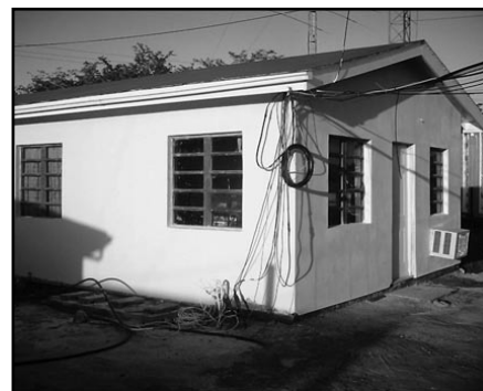
The V26B radio building
